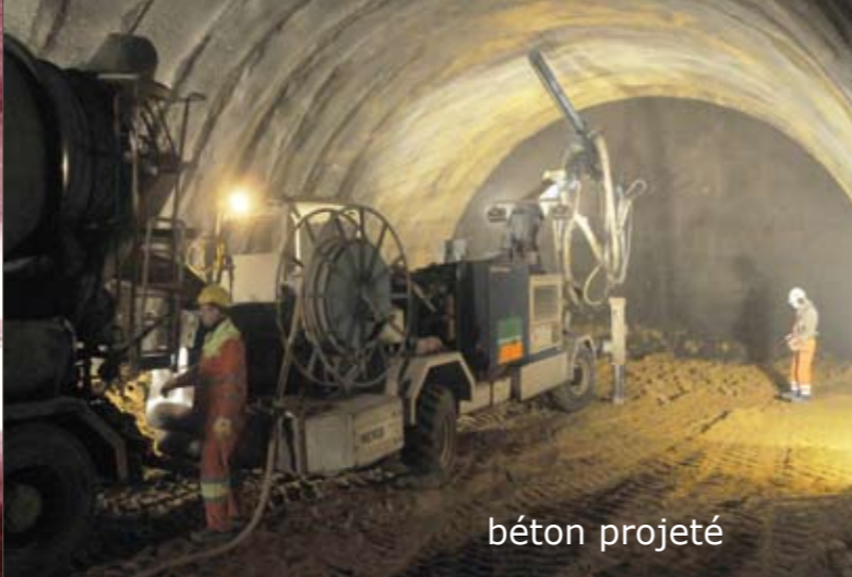
tunnel stafelter creusement
